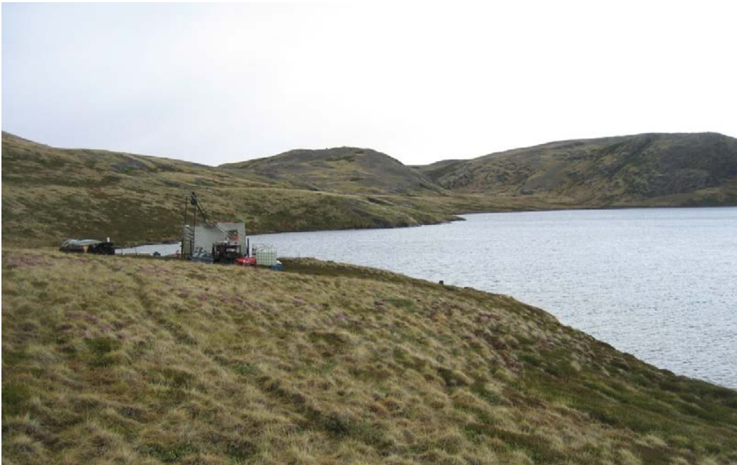
Figure 5-3. Drilling of DH-GAP01 to investigate the talik beneath the lake. The drilling direction is towards the lake. Photo by Timo Ruskeeniemi.
