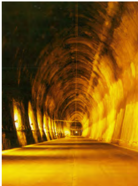
Figure 7-11. Typical JOGMEC underground rock cavern used for storing fuel oil. JOGMEC specifically notes that the design “...features high resistance to earthquakes...” (JOGMEC 2011).
