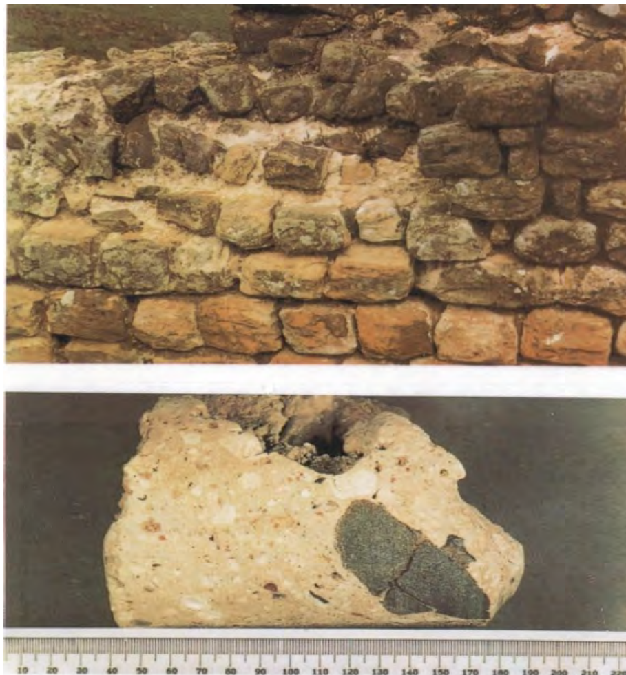
Figure 8-23. A close up of Hadrian's Wall (top) showing the mortar binding the stone blocks with (bottom) a section of core drilled through the wall (from Jull & Lees 1990).
