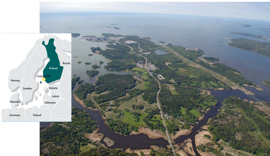
Figure 1-1. Olkiluoto Island is situated on the coast of the Baltic Sea in south-western Finland. Photograph by Helifoto Oy.
