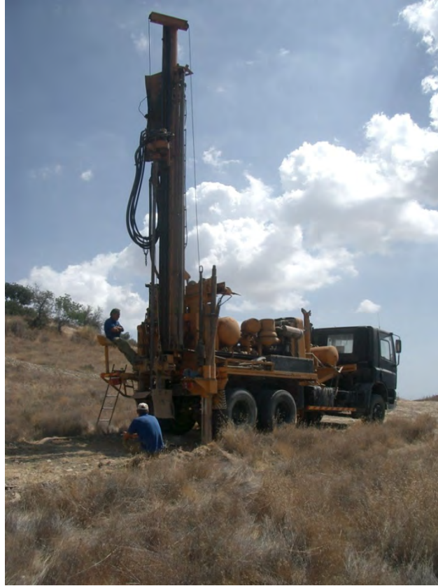
Figure 8-35. Drilling through the bentonite to access the reaction zone at the base. Parsata, Cyprus.
