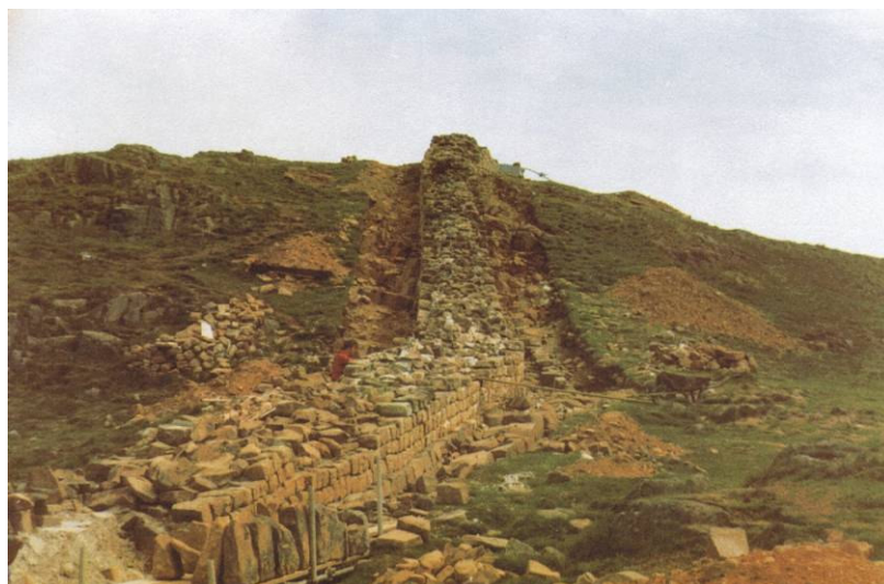
Figure 7: The remains of the 2000 year old Hadrian's Wall that includes cement mortars containing calcium-silicate-hydrate compounds.
