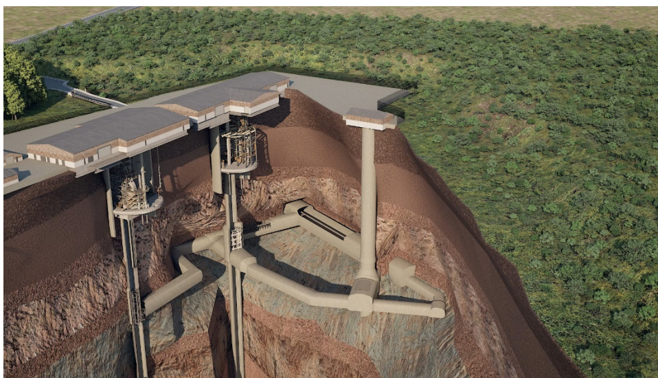
Figure 13.5-1. artists impression of the service (far left) and production (middle) shafts in the Woodsmith mine at Dove's Nest Farm, near the village of Sneaton, Yorkshire. Image courtesy Anglo-American plc.
