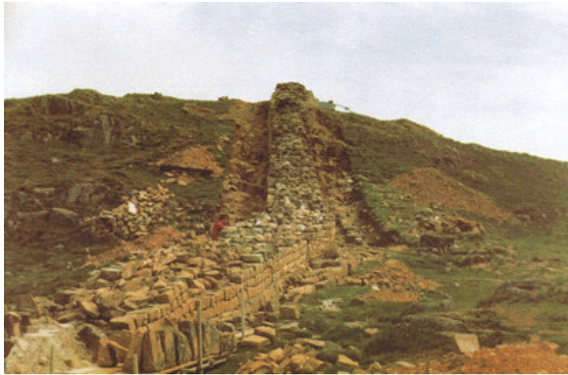
Figure 1 Section of the remains of Hadrian's Wall, showing the Romans' stone block construction bound together with cement (from Miller et al., 2000).
