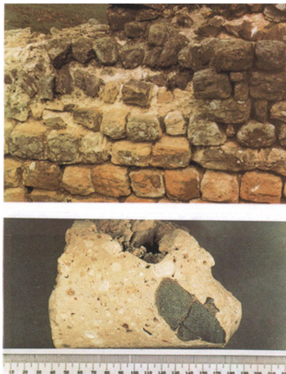
Figure 1 Section of the remains of Hadrian's Wall, showing the Romans' stone block construction bound together with cement (from Miller et al., 2000).
