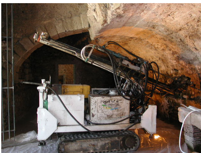
Figure 2: Left: drilling equipment installed in the internal gallery (ambulacrum). Right: Radial wall with masonry. (Photograph by I. Techer, GIS/CEREGE)
