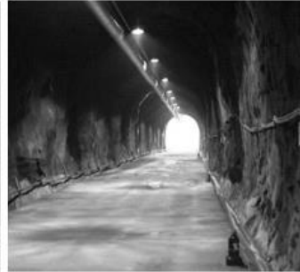
(b) Access tunnel
